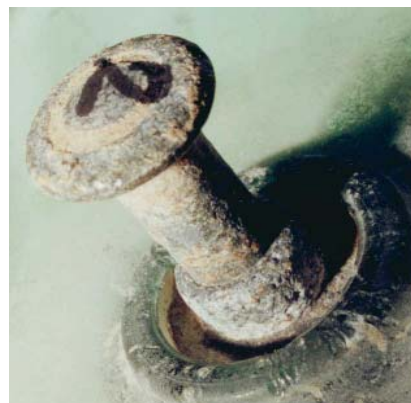
Figure 3: Zinc sleeve protection preventing and eliminating pin corrosion
