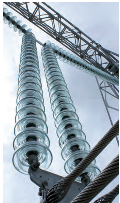
Vibration test for 800kV UHVDC TL at Bazet High Voltage laboratory, France
