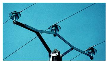
Pin type insulators for distribution lines, with an annual capacity of **700,000 units**
